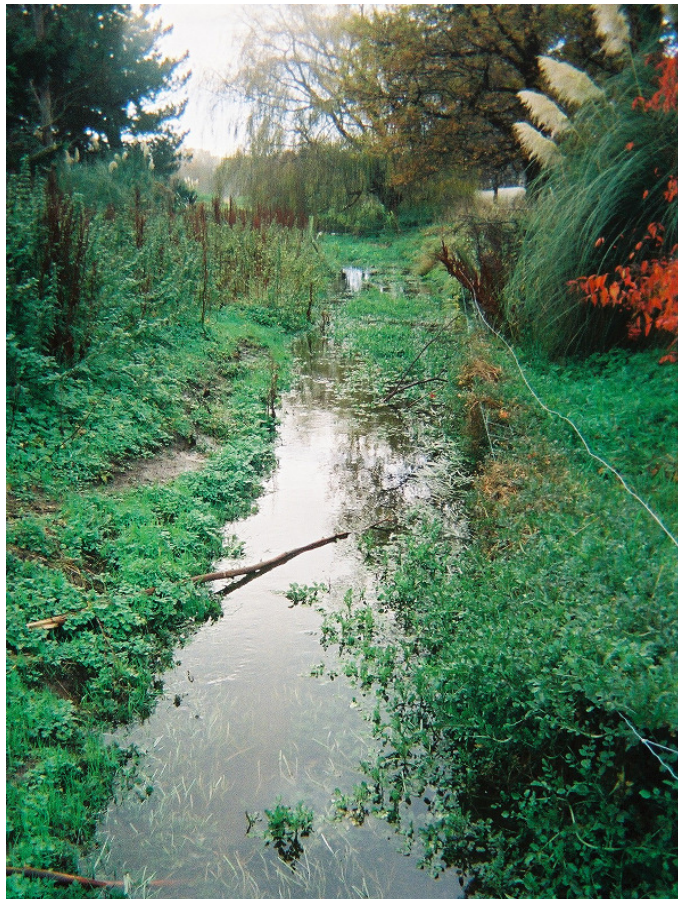
Figure 3.2: Drainage line downstream from Beach St Culvert
